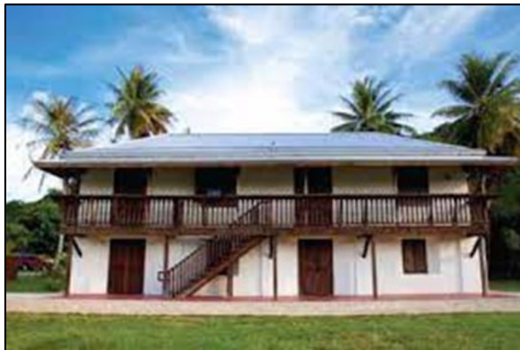
Figure 7. Historic Lujan House in Hågatña. Example of historic building that is listed on the NRHP. The house was reportedly built by hauling coral stones from Hågatña Bay and constructed via the CHamoru method of mampostería (stone and mortar). Photo Courtesy of the Guam Preservation Trust.
